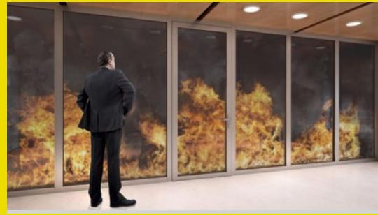
Insulation (I) is the ability of a component or construction to maintain the integrity of the element on one side only, without spreading the fire as a result of a significant heat flow from a heated side to a non-heated side. During the fire, the construction on the non-heated side reaches a temperature of not more than +140°C up to +180 °C.
