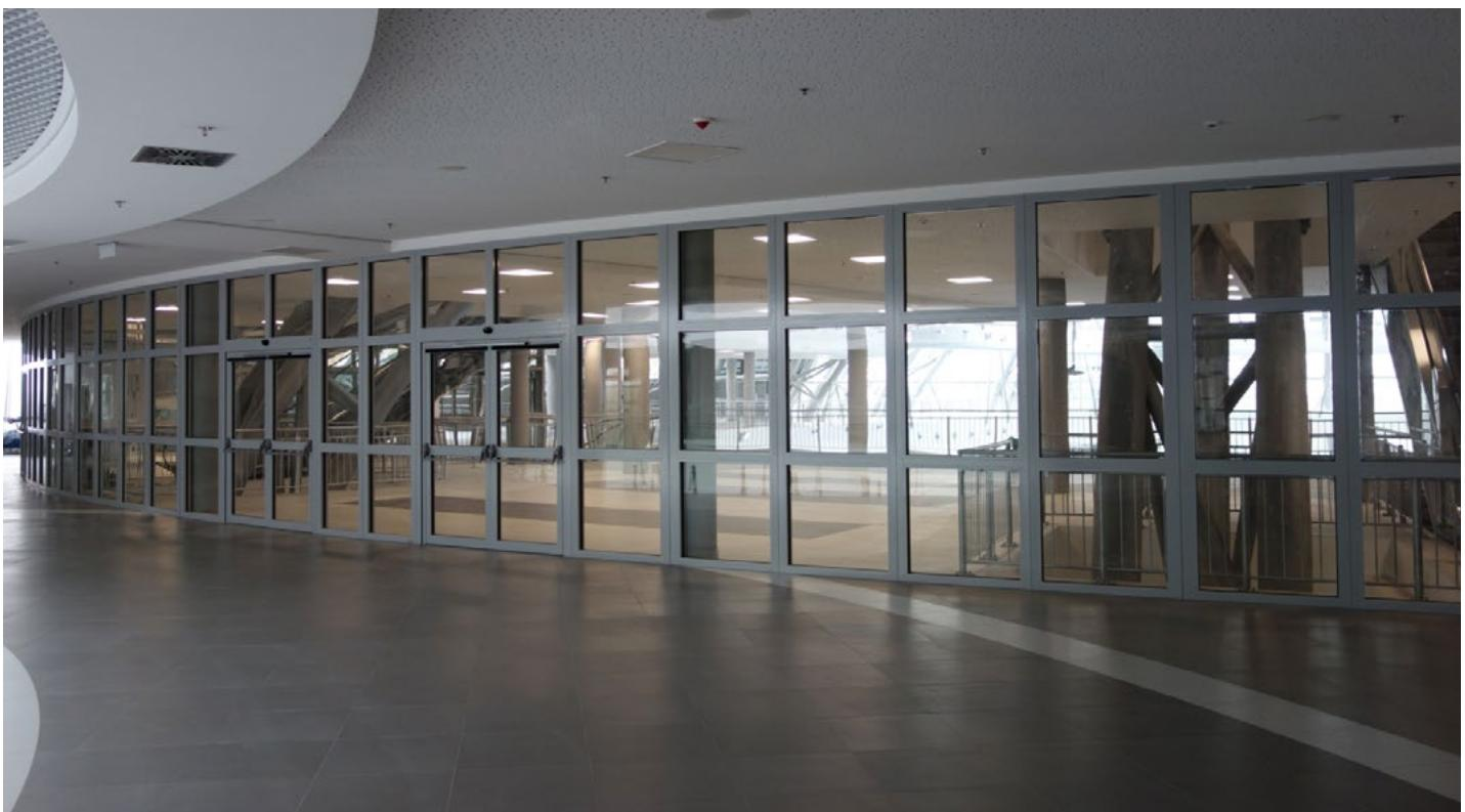
The **MB-118 EI** fire rated walls are used to make fire partitions with fire resistance class of EI 120. The system is classified as non-fire spreading (NRO). Its design & construction is such that, it provides a technical connection with the **MB-78EI** door, which means a number of common components (such as glazing beads, cooling inserts, expanding tapes, seals and most accessories) and also similar to the basic system, production and installation technology.
