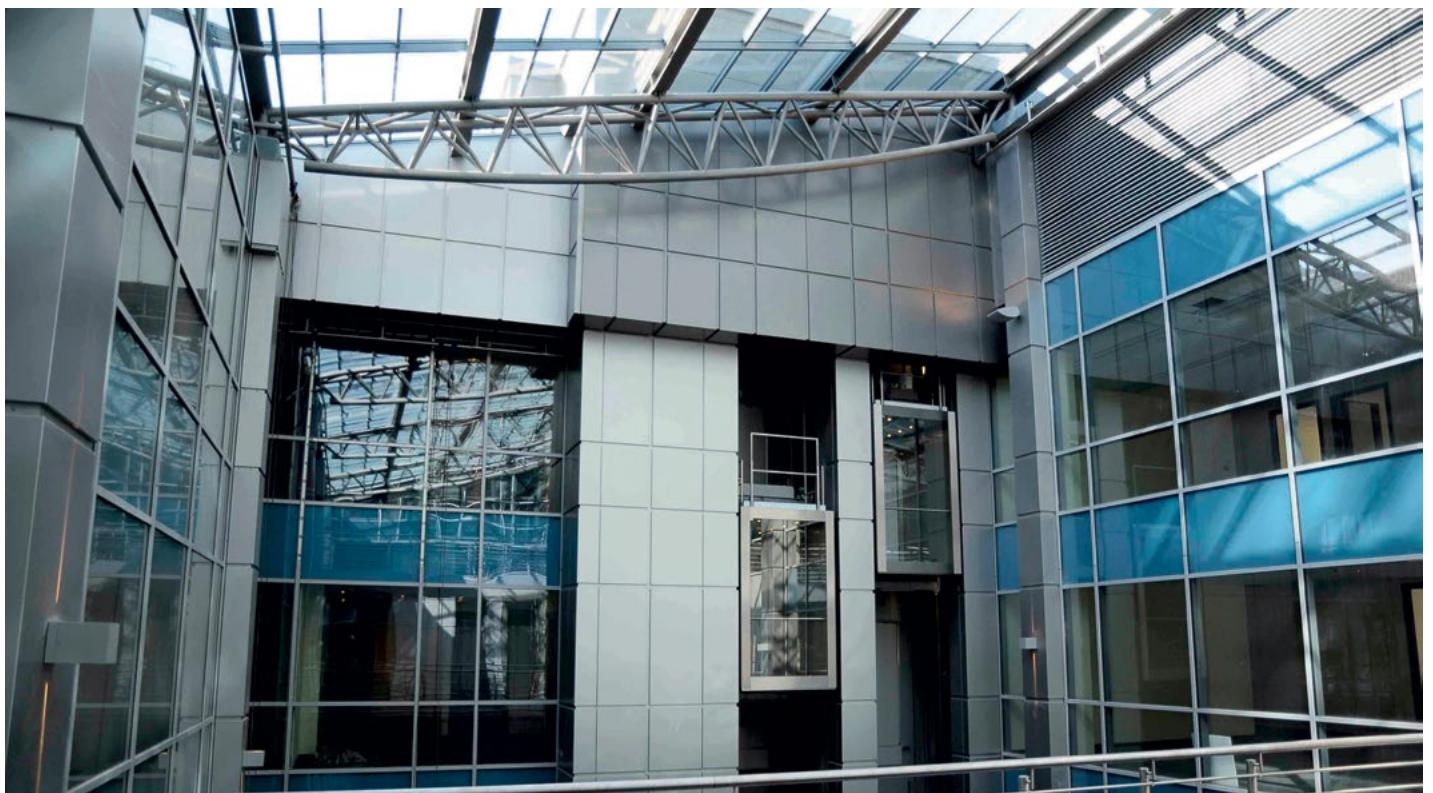
The **MB-SR50N EI** curtain wall fire rated systems have been developed to provide a light-weight curtain & fire resistant wall, of classes EI30, EI60 classes according to PN-EN 1364-3 and PN-EN 1364-1 and of fire-resistant glass-covered roofs. The system is classified as non-fire spreading (NRO).
