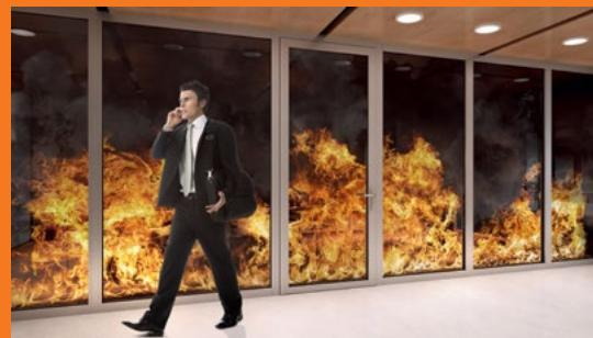
Reduction of radiation (W) is the ability of a component or construction to maintain the integrity of the element on one side only, to reduce the likelihood of fire spreading that may result from significant thermal radiation or through an element, or from its non-heated surface to adjacent materials.
